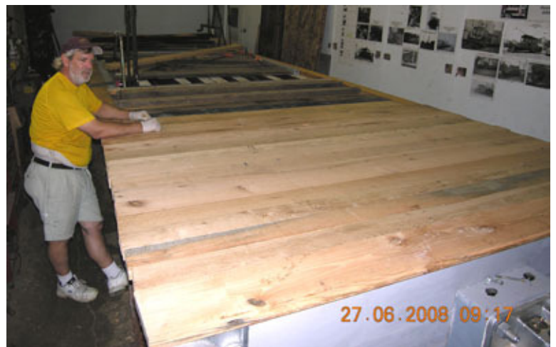
No. 1 end deck fitted
