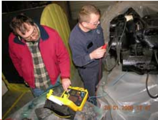
Roger Paradie preparing to test the insulation resistance of one of 100’s motors at A. C. Electric Using STM’s new AEMC 1,000 volt megger.
