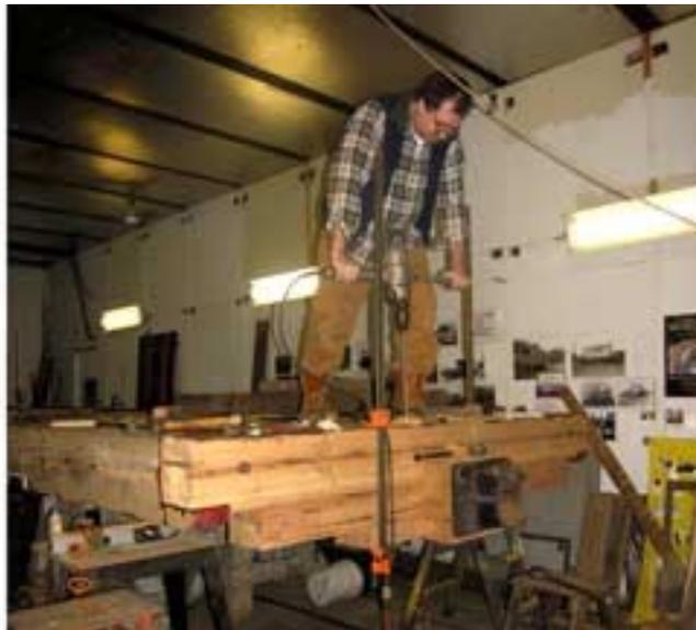
Randy Leclair using the big drill to make holes for bolts to fasten sill assembly together.
