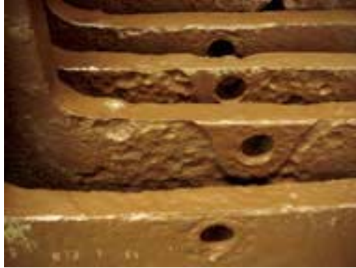
Pitting around the bolt holes for the spring seats on the equalizer bars
